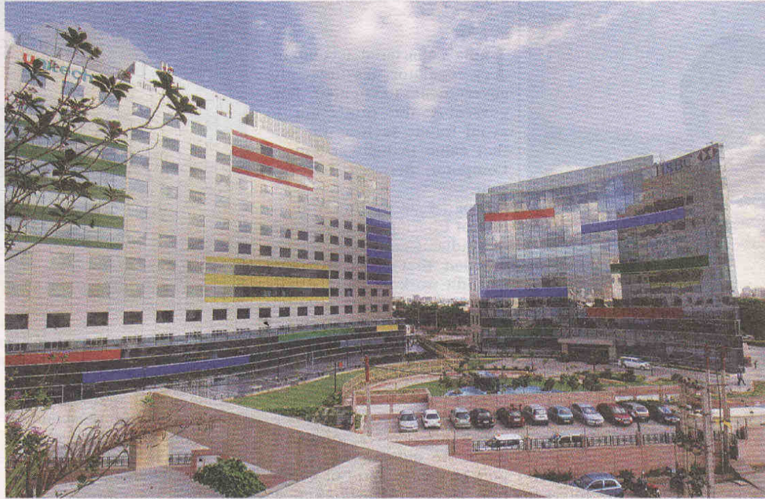
New initiative: The Unitech and HSBC offices in Gurgaon, which have been certified as green buildings. BEE plans to ask developers to build a model green flat, with energy-efficient features.
